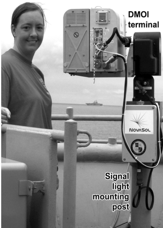
Figure 5: An existing signal light was removed and its mounting post used for installation of the DMOI terminal on the host vessel
