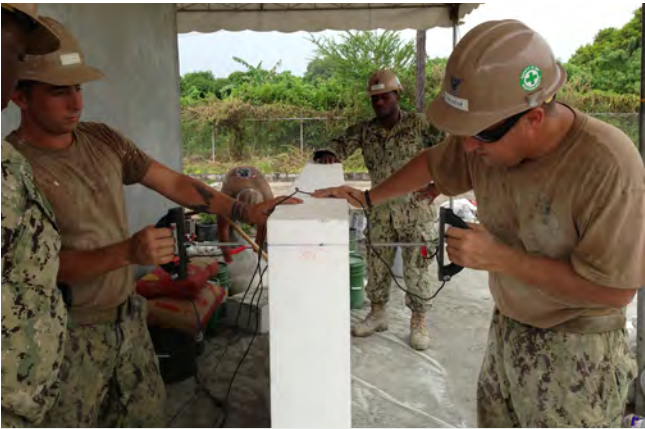
Seabees construct a building in the Philippines using specially treated Styrofoam that allows the structure to withstand typhoon-force winds. Photo by Dave Collier
