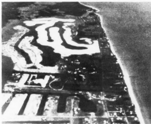
Figure 8 - Land reclama- tion near Na- ples, Florida.
