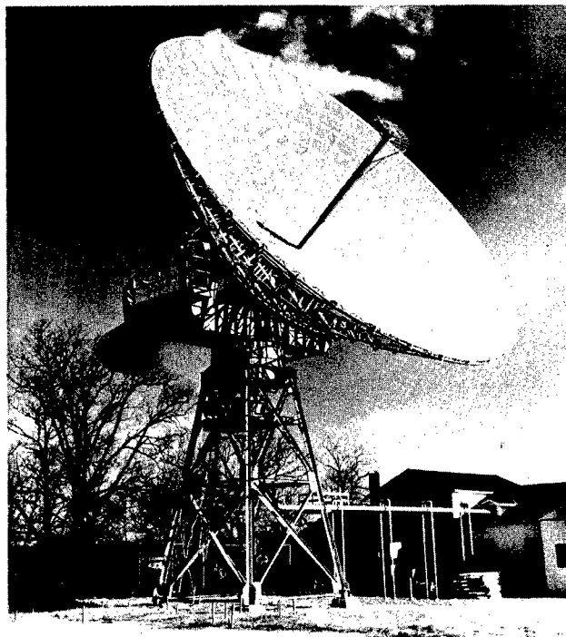
The Diana radar transmitter, Fort Monmouth, New Jersey.
