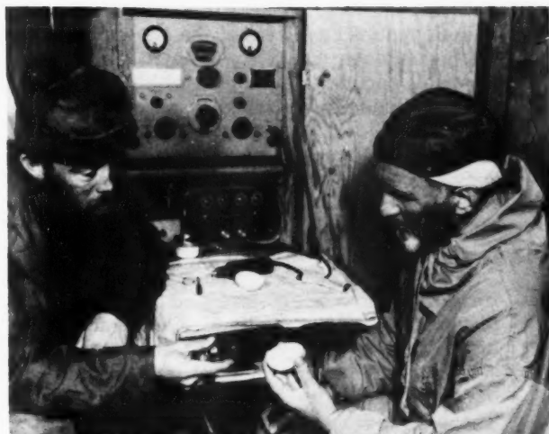
Charlton, left, displays temperature telemeter which has been prepared for insertion in penguin egg shell held by Eklund.
