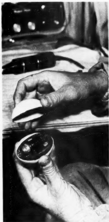
The radio thermometer and empty penguin egg shell are readied for use. Left, the telemeter is placed in shell. Right, albumen is injected into sealed shell.
