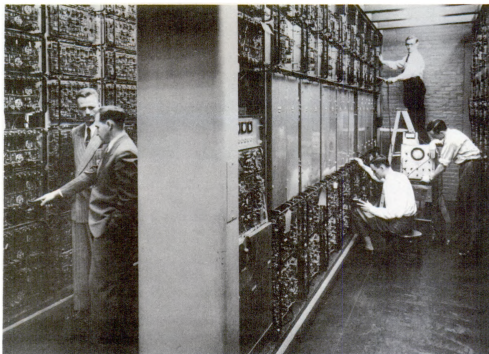
Figure 1--Central computer unit of Whirlwind I occupies 224 lineal feet of racks, ten feet high.
