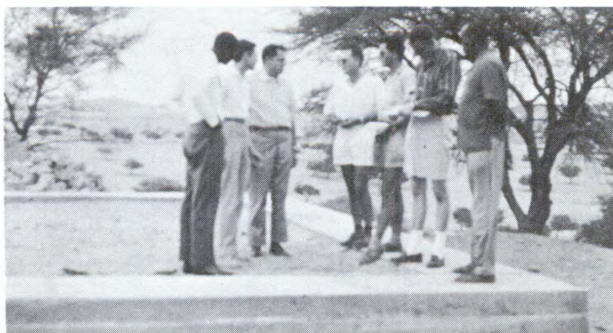
Site at Boure was built on foundation of unfinished building. Here crew inspects with local officials.
