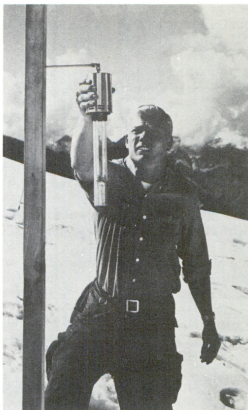
An IGY glaciologist reads a precision psychrometer to determine relative humidity over the McCall Glacier, Alaska.
