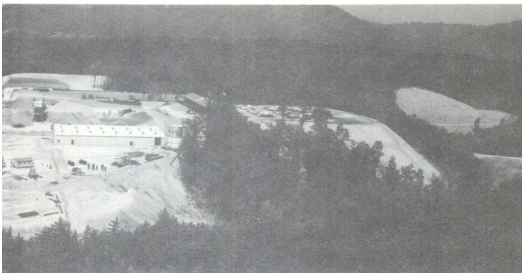
above, panorama of the site for the Naval Radio Research Observatory near Sugar Grove, W.Va. The 600-foot radio telescope will be mounted in area at left side of photo behind tank.
