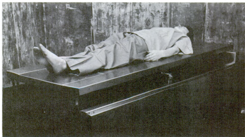
Patient in position on the plastic-crystal, whole-body radiation counter in the "quick and dirty" room.
