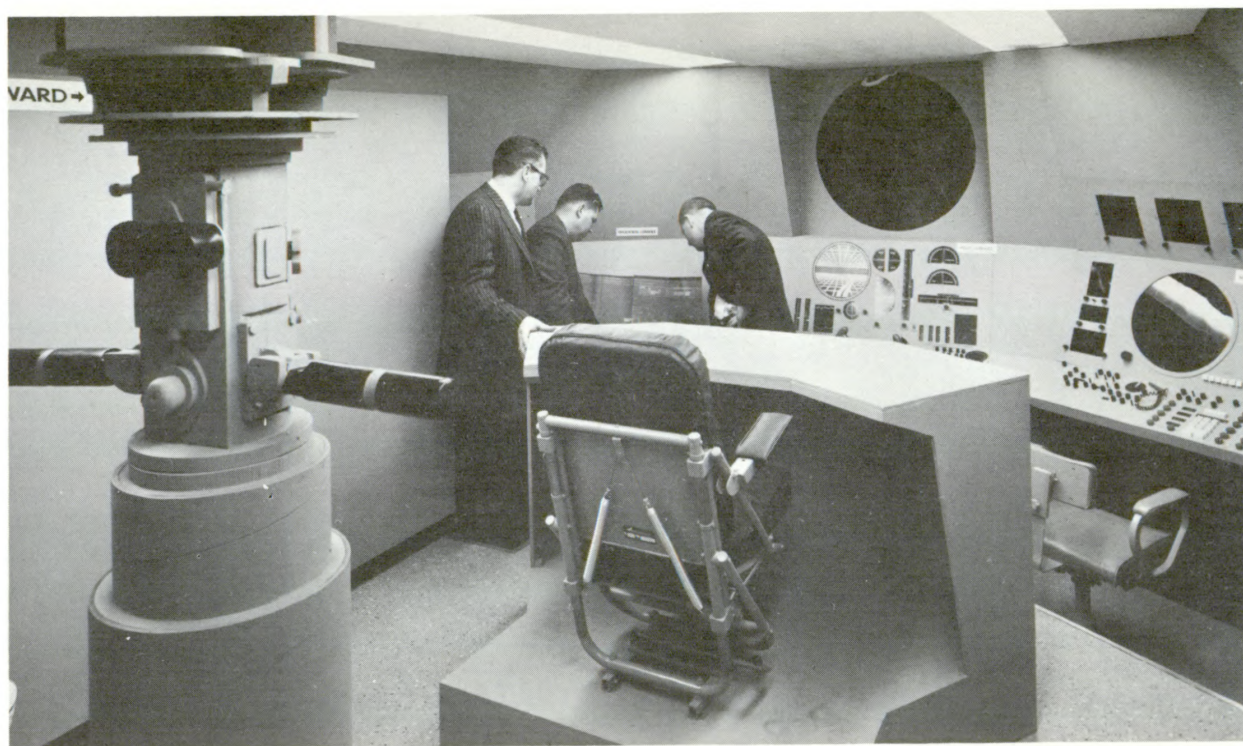
Mockup of an integrated control center for nuclear submarines of the near future. These simplified controls utilize electronic computers, data-processing equipment, and visual displays. They are the results of SUBIC (integrated control applied to submarines), which combines the control of five fundamental submarine systems – weapons, communications, engineering, ship, and environmental. Note the absence of cable network. Coordinator of SUBIC's Navy-industry contractors, is General Dynamics Electric Boat Division, Groton, Conn. (General Dynamics photo. )
