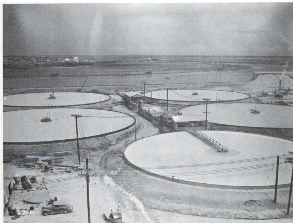
Figure 3 - Magnesium hydrate is precipitated in these tanks by the addition of lime or caustic to sea water in the Dow Chemical Company facilities in Freeport, Texas. (Courtesy of Dow Chemical Co.)
