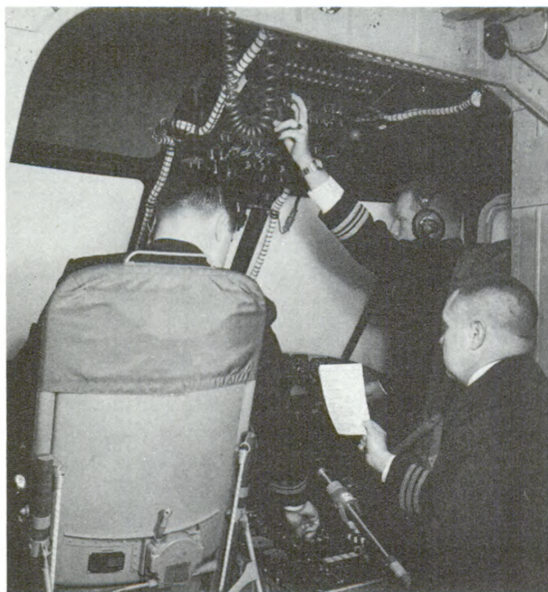
The "cockpit" of the new HSS-2 helicopter flight and weapons simulator.
