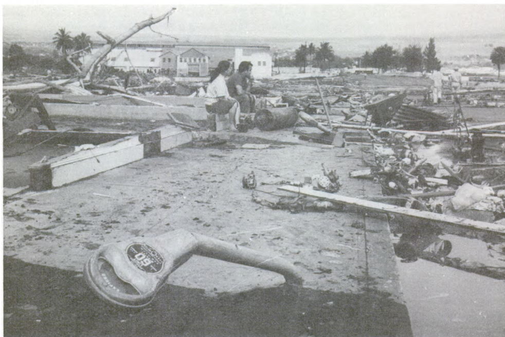
Tsunami damage at Hilo, Hawaii. (Photo courtesy of The Honolulu Advertiser .)
