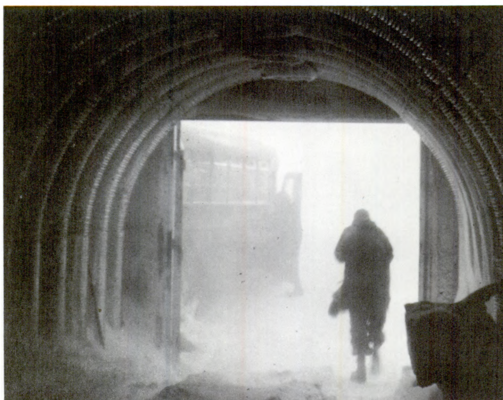
Entrance to tunnel; Phase I weather conditions outside.
