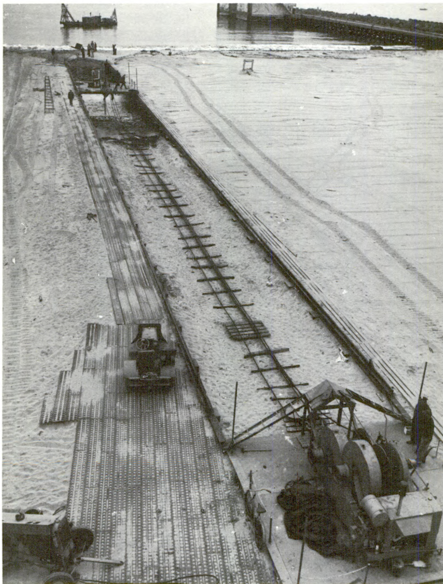
The anchor-testing facility at Port Hueneme
