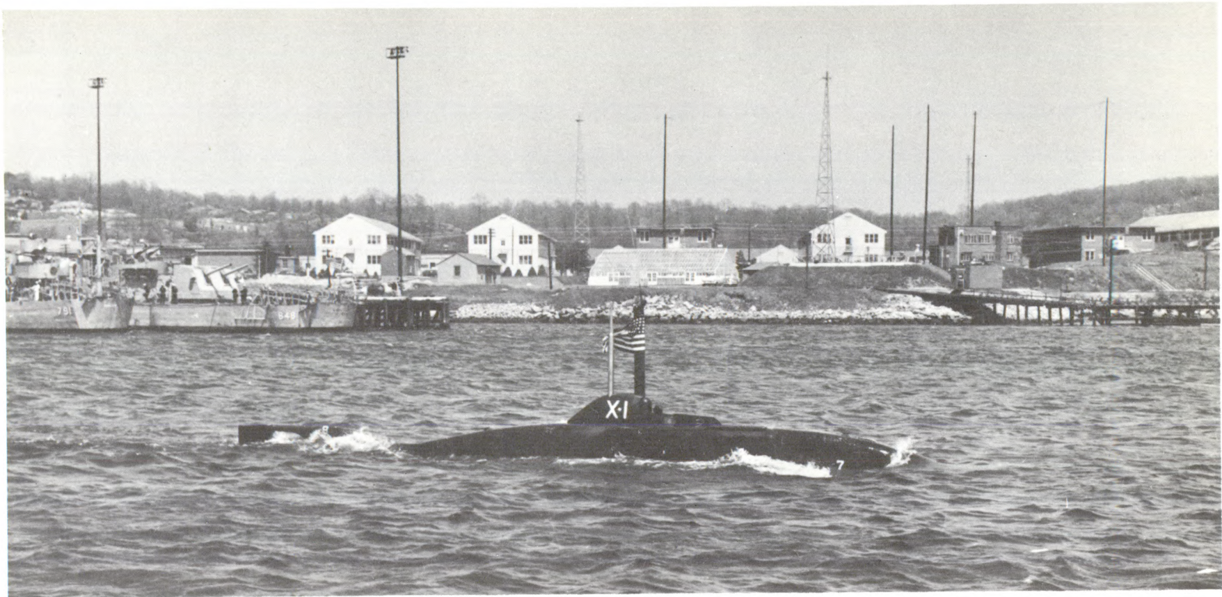
This experimental midget submarine, SS X-1, is solely a research vessel. Like the TRIESTE, described elsewhere in this issue, the X-1 is one of the specialized vehicles being used in the Navy's broad program of oceanographic research. The boat is presently operating in the Chesapeake Bay.
