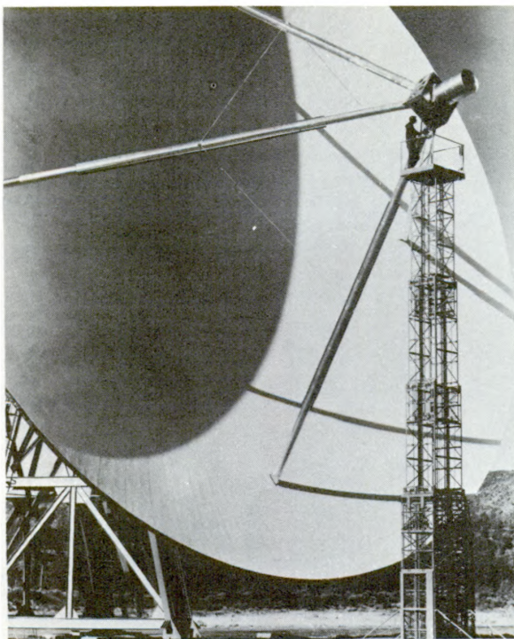
Atop portable elevator a technician makes adjustments on the antenna "horn" at focus of the new 85-foot telescope. Radio waves are reflected into the coaxial horn, then sent to receivers in a laboratory building nearby.
