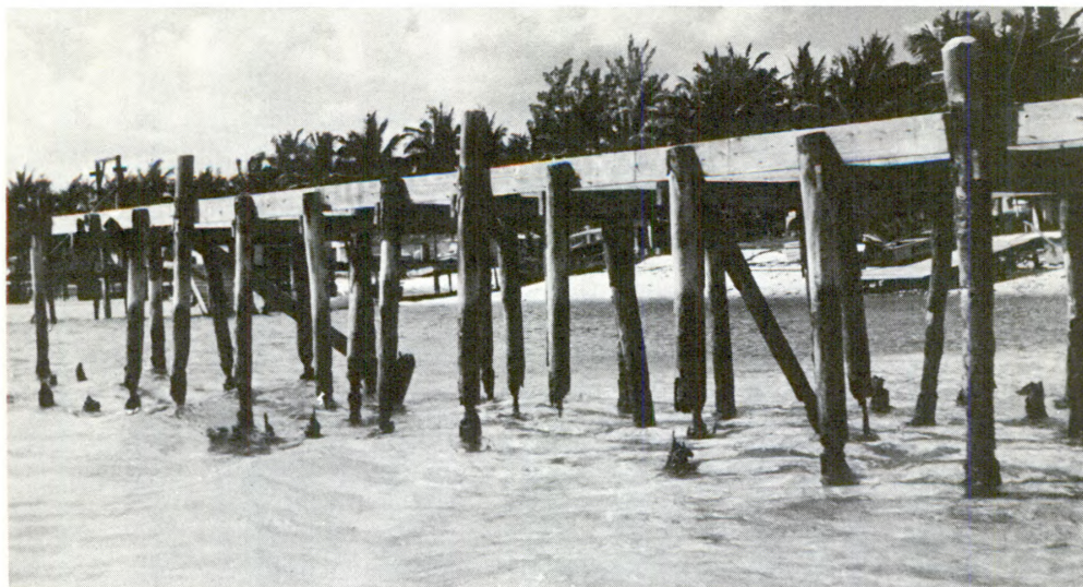
Biological deterioration of wood pilings.
