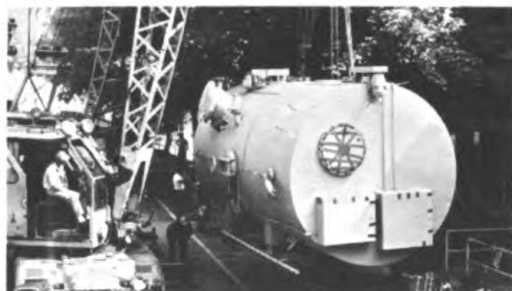
The Climate-Altitude Chamber in process of installation at MRL in July 1963. The tank weighs 25 tons. Its inside dimensions are 9 feet by 9 feet by about 7 feet (height).
