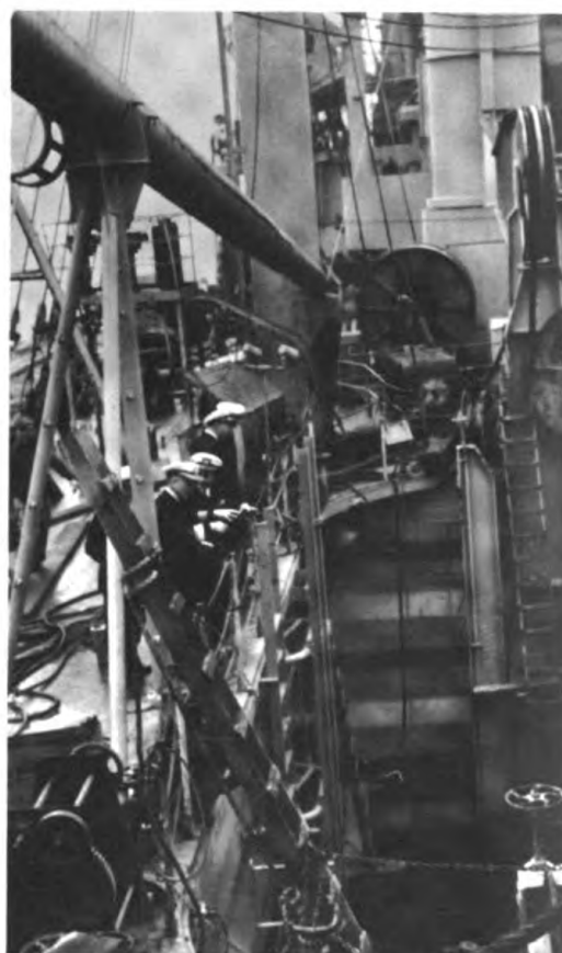
Inspection party views the well through which the sound source is lowered.
