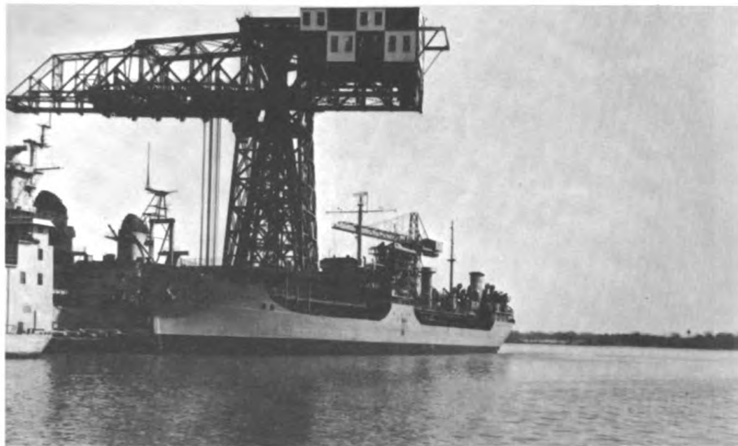
The USNS MISSION CAPISTRANO moored under the large hammerhead crane at the Philadelphia Naval Shipyard. This crane is one of the few facilities in the U.S. capable of handling the Artemis multi-hundred-ton sound source. ● ●
