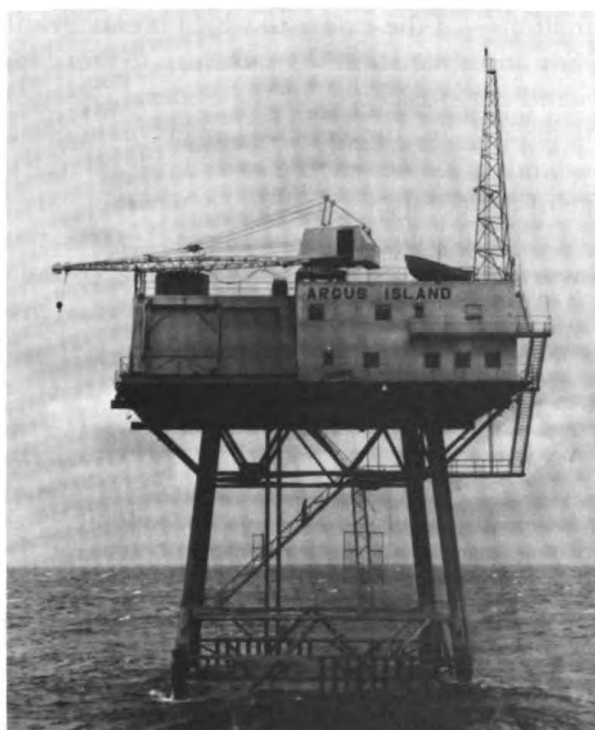
Research tower ARGUS ISLAND erected by the Navy 30 miles southwest of Bermuda
