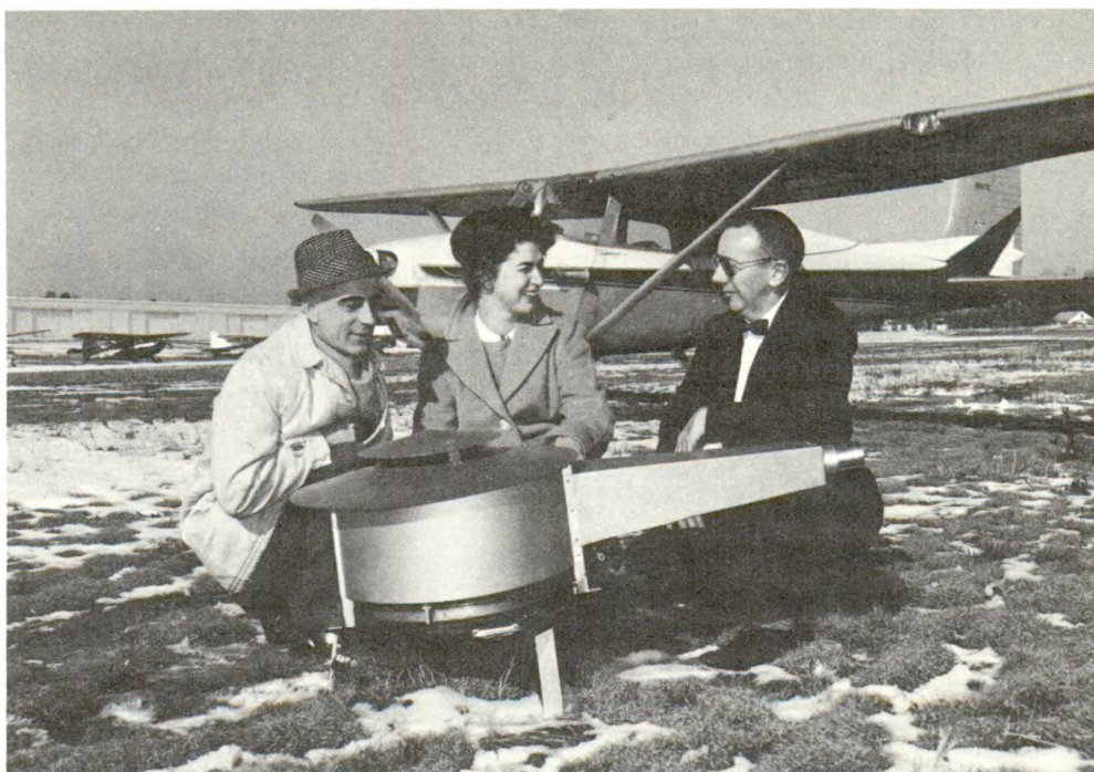
Figure 4 — Alan W. Baldwin, Barbour Lee Perry, and Henry P. Birmingham, co-inventors of the Rainbow Optical Landing Aid, discuss the performance of an experimental unit during one of the preliminary field tests conducted with light aircraft last winter.
