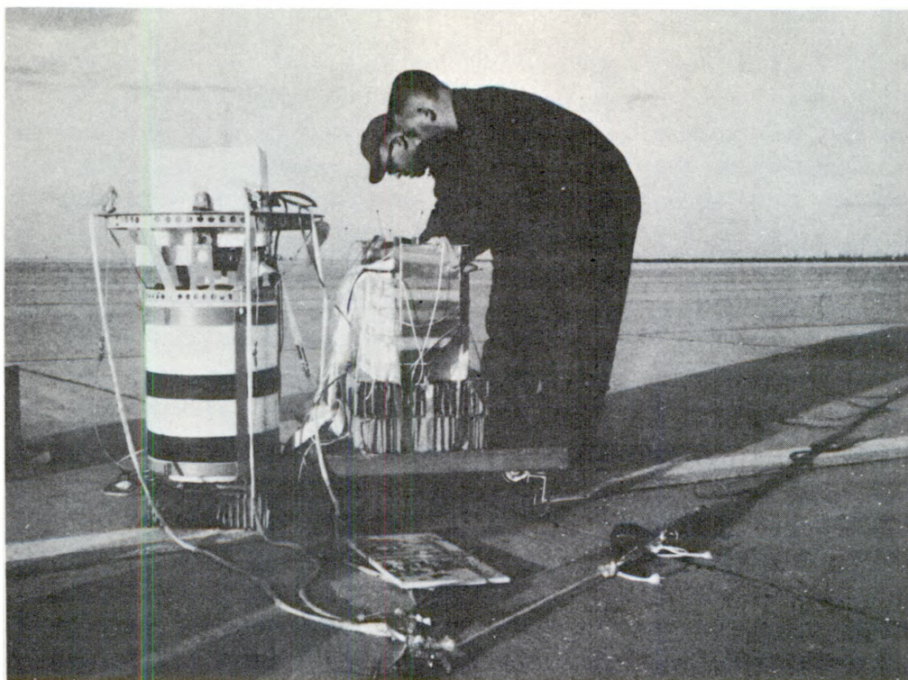
Technicians prepare flight payload for NRL cosmic-ray experiment. The stack of nuclear emulsions is located in the white box at the top of the gondola.
