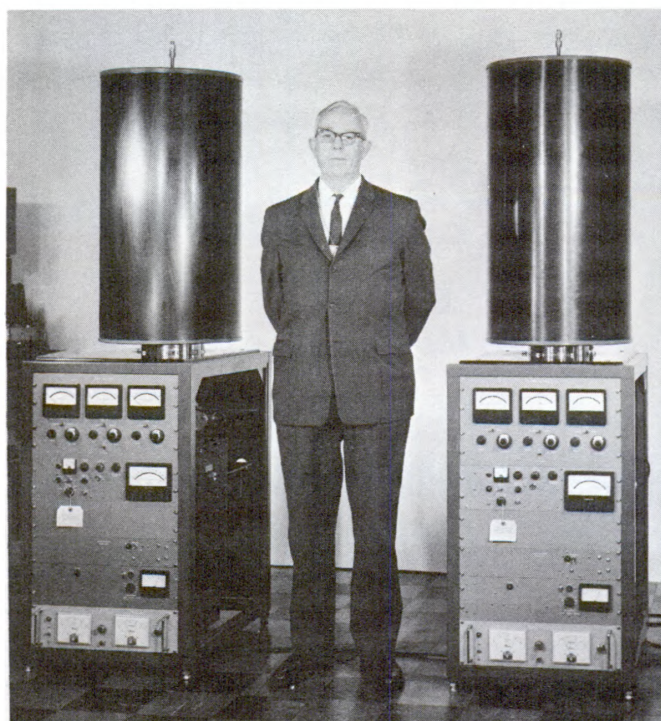
Figure 4 — Atomic hydrogen masers. The units were built by Bomac Laboratories under contract to ONR and evaluated and used by the Naval Research Laboratory.
