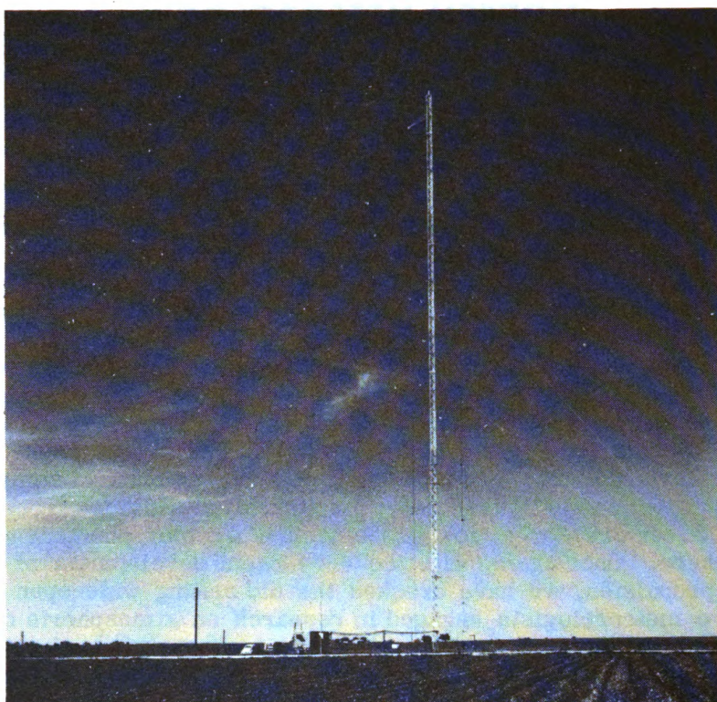
Fig. 9. General view of the 300-ft meteorological tower of the Electrical Engineering Research Laboratory, University of Texas. This tower is located about 15 miles northeast of Austin, Texas, on a gently rolling cottoncultivated terrain. Instruments for measurement of temperature, moisture, and wind gradients are strung from booms at top of tower.
