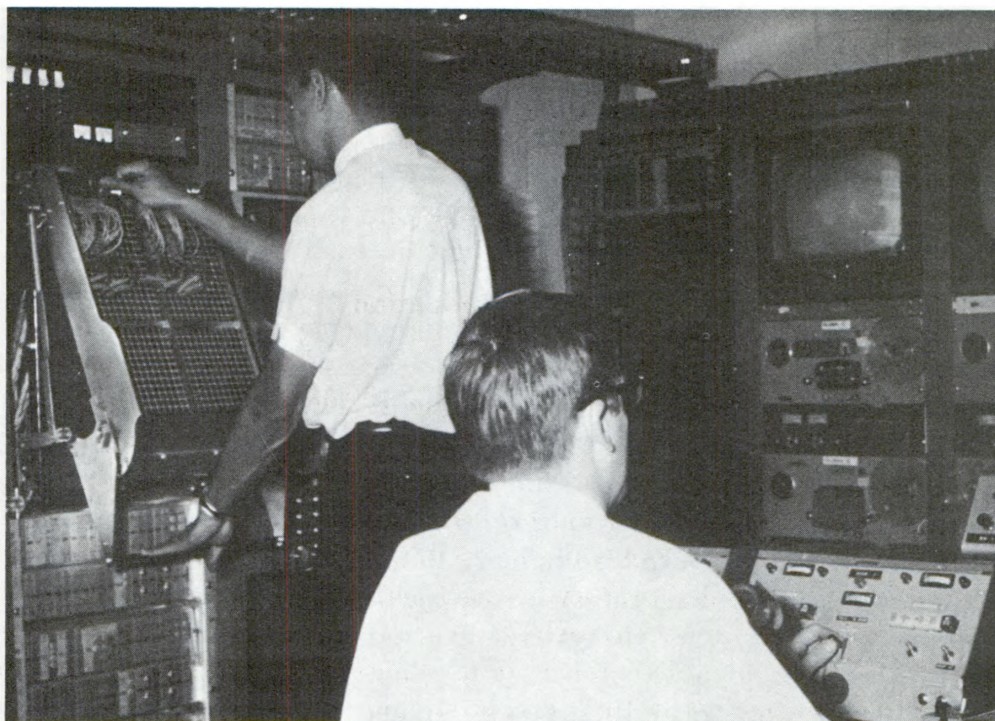
Monitors in the central experimental control room
