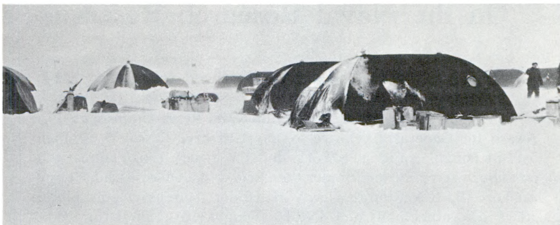
The huts on the Soviet station were made of insulated canvas stretched over frames to form hemispherical structures
