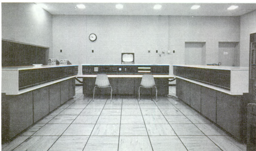
Figure 2 — Front view of the VCAD generator as installed in the Naval Missile Center's Advanced Display/Control Evaluation Laboratory
