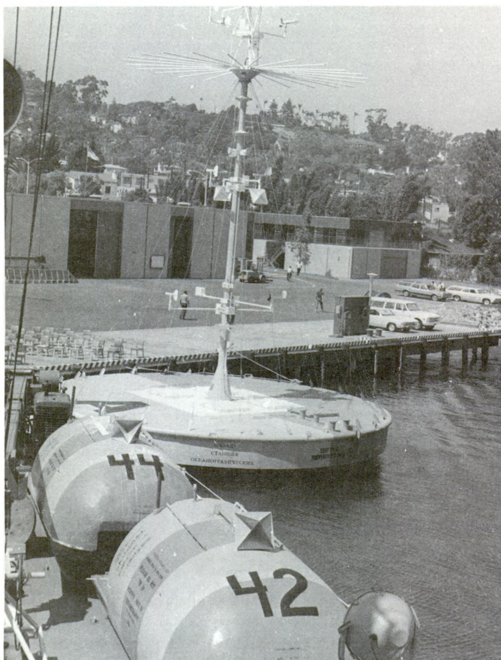
Bumblebee buoys and monster buoy Alpha awaiting to be transported to the North Pacific Ocean. Both types of buoys have been tested in the ocean and have survived 100-mile winds and 45-foot waves.
