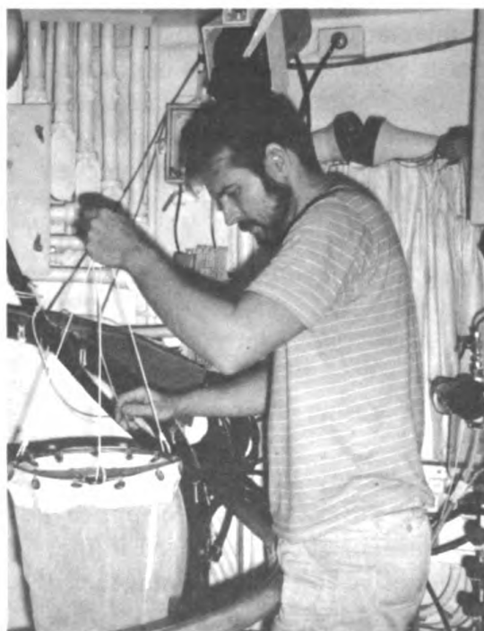
Richard Waller changing an auxiliary CO 2 "scrubber" in the life support and environmental control systems
