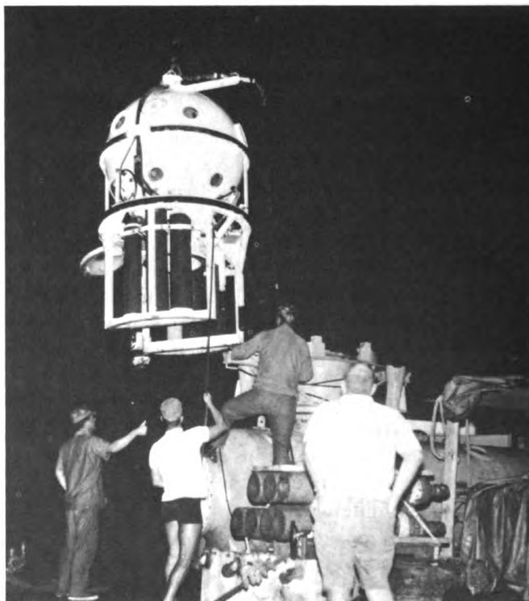
On April 15 between 12:15 and 12:45 AM the aquanauts surfaced. The personnel transfer capsule brought the aquanauts from the Tektite habitat to the decompression chamber in groups of two.
