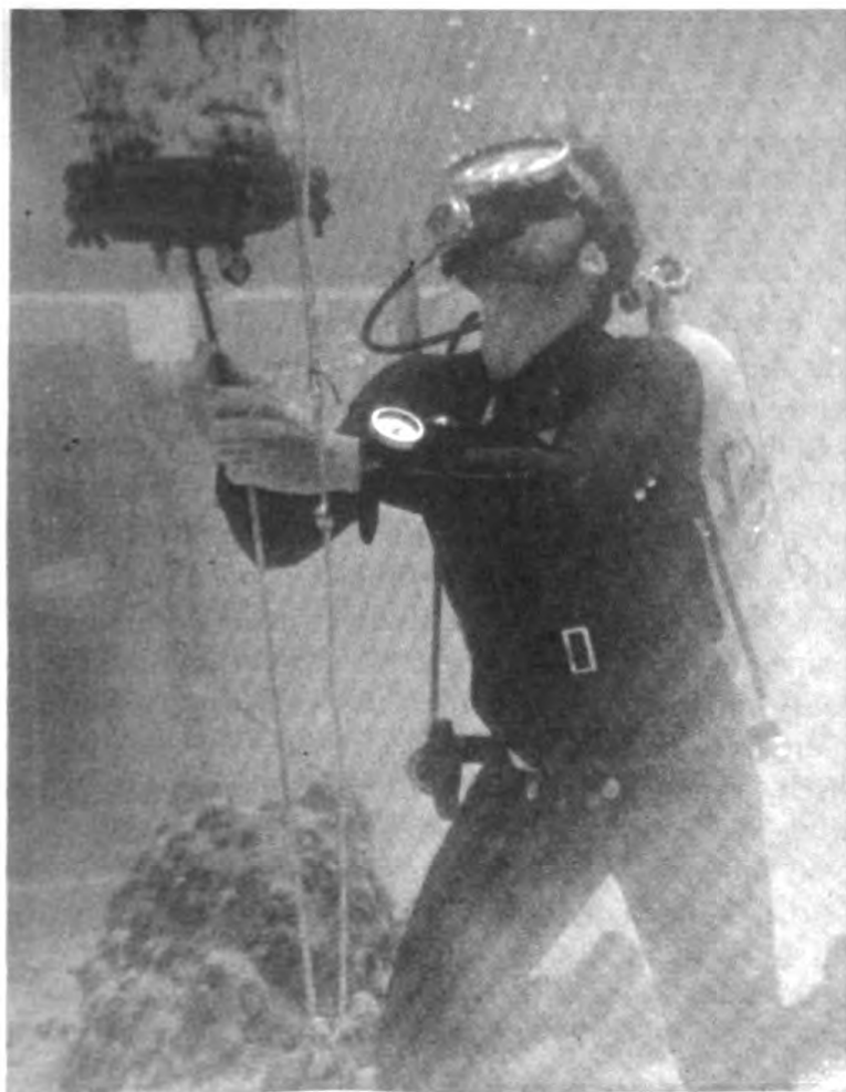
The aquanauts used transfer pots as pictured here to receive and send equipment to the surface
