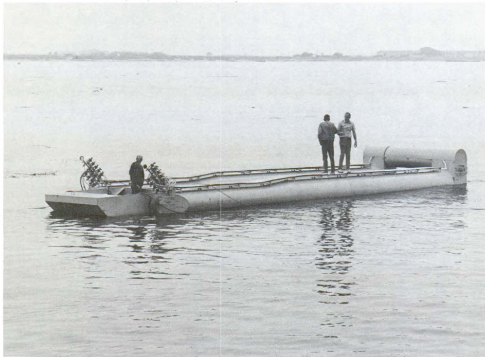
Figure 2 — A two-legged, one-eighth scale, operational module, some 42 feet long, is tested in San Diego Bay by UCSD's Scripps Institution of Oceanography personnel during feasibility studies. Eventual construction of a full-scale module whose 350-foot concrete legs, when extended vertically in the ocean, would provide stability for a floating platform. Additional modules could be linked to form platforms of any size desired for oceanographic research in the deep ocean.
