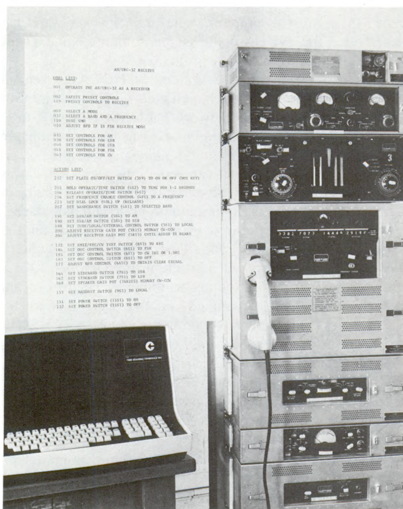
Figure 1 — Student station for TASKTEACH. Student interacts with a TASKTEACH program via keyboard-display terminal at lower left. Apparatus at right is AN/URC-32, on which student is learning to troubleshoot. List on upper left is for student's constant reference.
