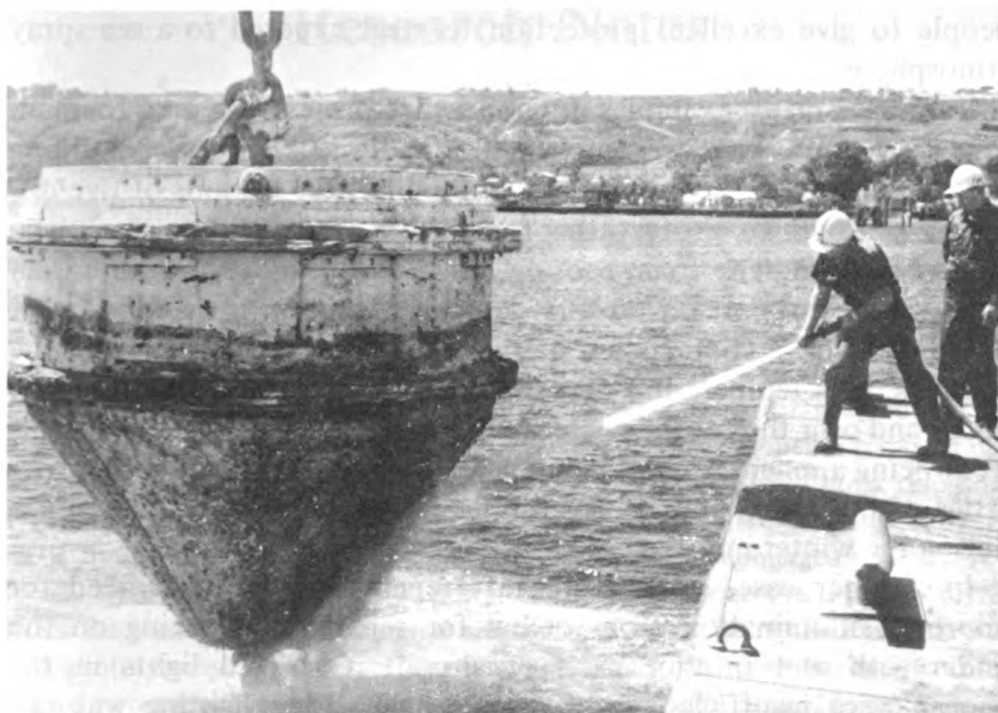
Figure 5 — A mooring buoy with an experimental protective coating is washed down for an annual inspection
