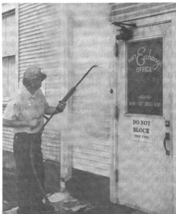
Figure 3 – A steam cleaning system was evaluated during the investigation of new and improved methods for cleaning and maintenance painting of Navy structures
