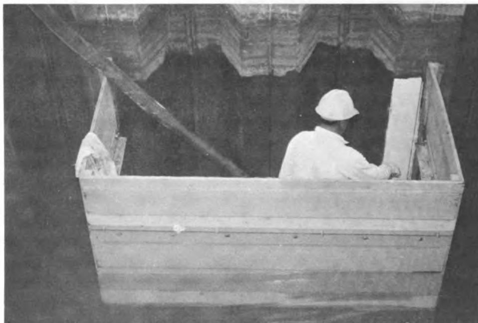
Figure 2 – The CEL cofferdam permits sand blasting and maintenance painting of steel piling to 2 feet below the mean low water mark
