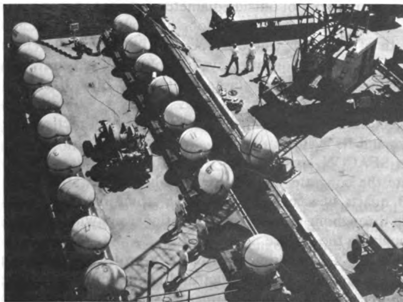
Figure 5 — These eighteen 66-inch outside diameter concrete spheres are currently undergoing long term testing in the ocean at depths between 2000 and 5000 feet
