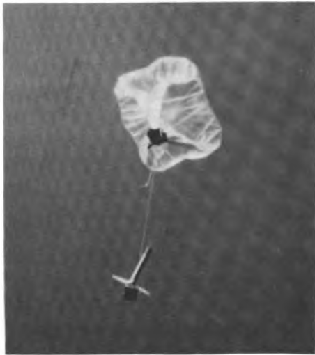
Figure 3 — Project ROCKOON in the early 1950's involved the launch of sounding rockets from small balloon platforms at an altitude of about 20 km.
