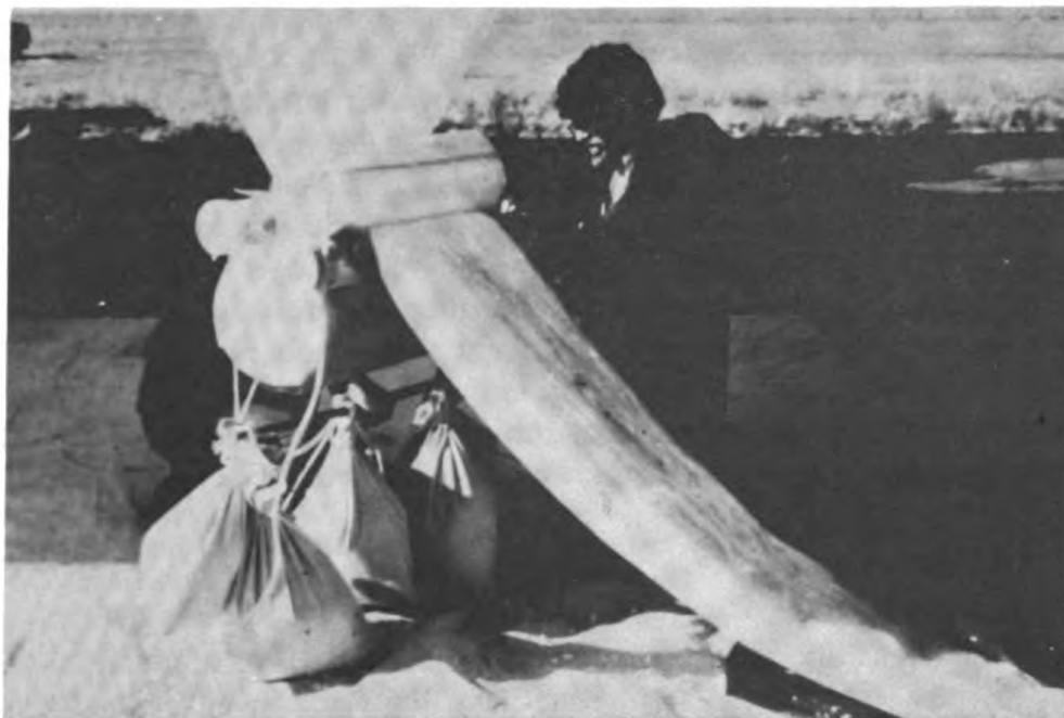
Figure 8 — Bubble restraint mechanism developed by University of Wyoming group. This device has been successfully employed in launching gross inflations of up to 260 lbs. .
