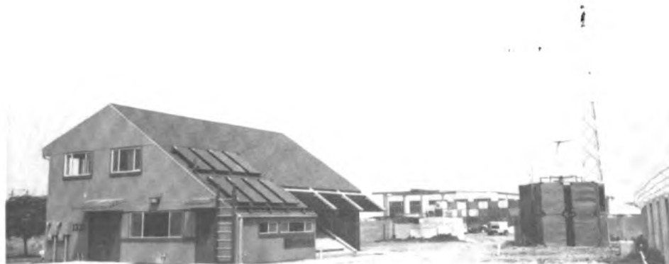
Test bed for energy research — The Advanced Energy Utilization Test Bed (AEUTB) at the Navy's Civil Engineering Laboratory, Port Hueneme, Calif. is the only system designed and fabricated solely for research and development of energy conservation and alternate energy sources.
