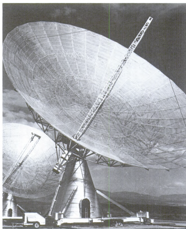
Giant twin radio telescope, located in the Owens Valley, 260 miles from Los Angeles, was built in 1959 by the California Institute of Technology with funds from ONR. During the first two months of operation, the telescope located and identified nine new radio sources outside our galaxy. Working in tandem, the 90-foot dishes produced a resolving power greater than any radio telescope of the day; that is the ability to pinpoint radiating objects in space. During the formative years of radio astronomy, ONR was the major sponsor in the United States. The Owens Valley telescope was one of several built and operated with ONR funds during the 1950's through the 1960's.
