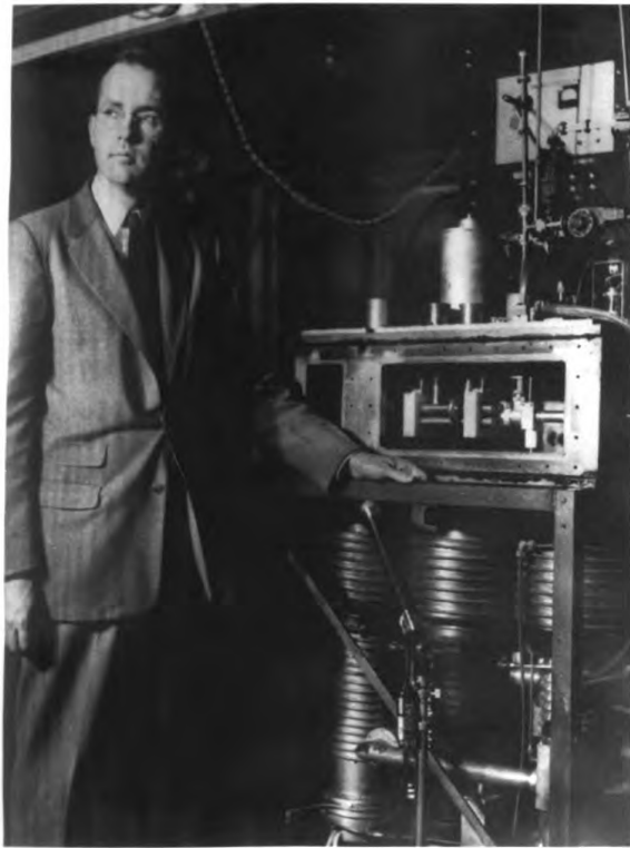
Professor Charles H. Townes is shown with the ammonia beam maser he developed in the early 1950's at Columbia University. This was the first molecular oscillator and amplifier and led to the development of the general field now called quantum electronics. This research was funded by ONR, the Army, and the Air Force.
