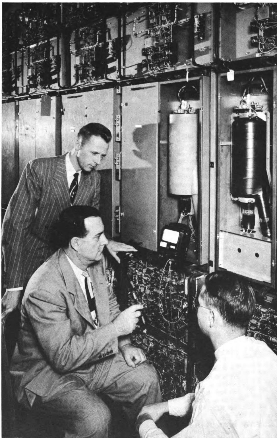
Here is what Whirlwind I's "memory" looks like. Electrostatic storage tubes enable the machine to "remember" information in less than one twenty-five-millionth of a second. Shown testing a tube assembly are Jay W. Forrester, Director of the Digital Computer Laboratory, Patrick Youtz, Head of Storage Tube Development and Stephen H. Dodd, Jr., in charge of systems engineering.
