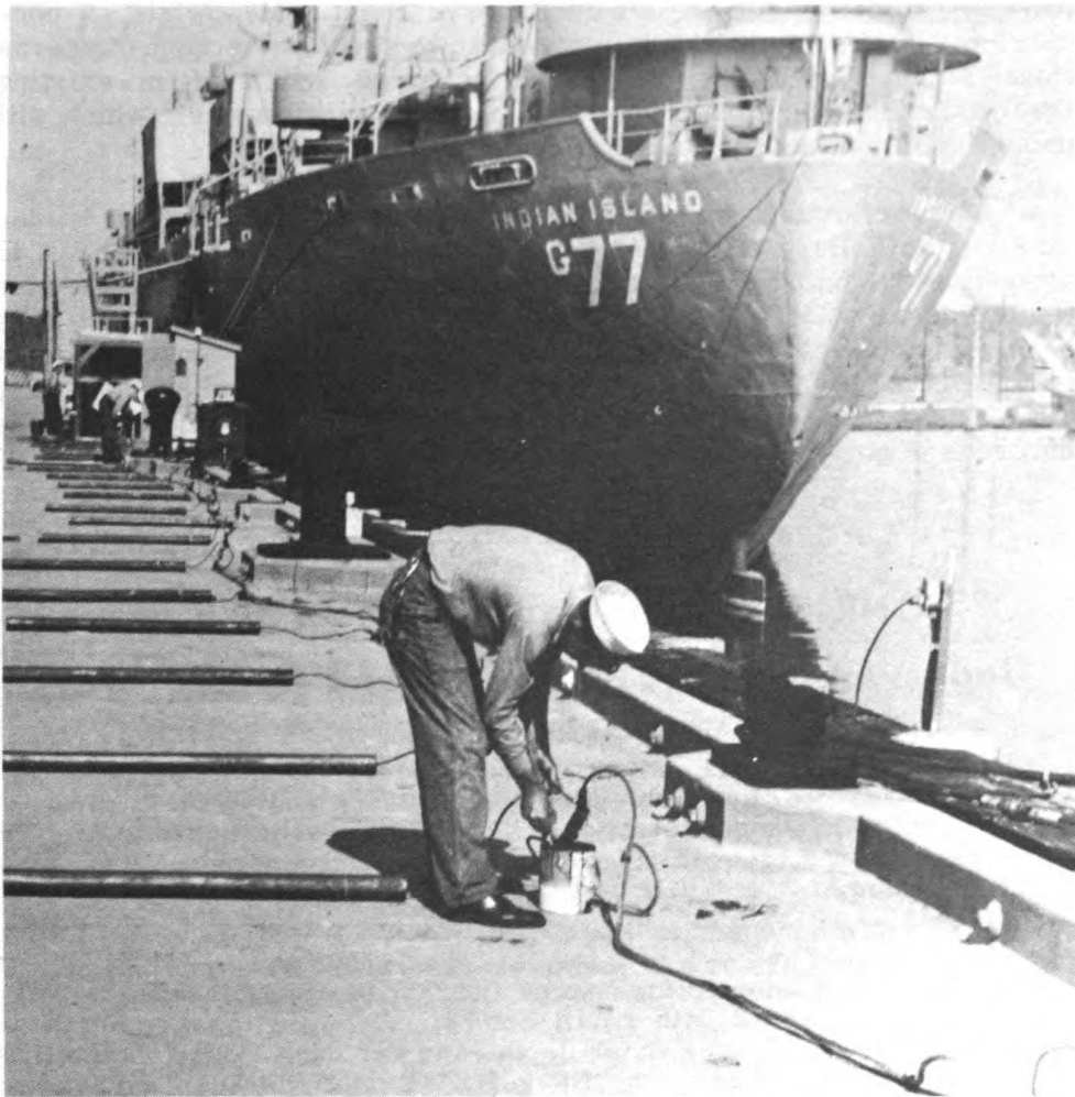
Figure 7. Attaching electrical cables to impressed-current electrodes. These graphite rods will be buried in the mud some 400 ft from the ship.
