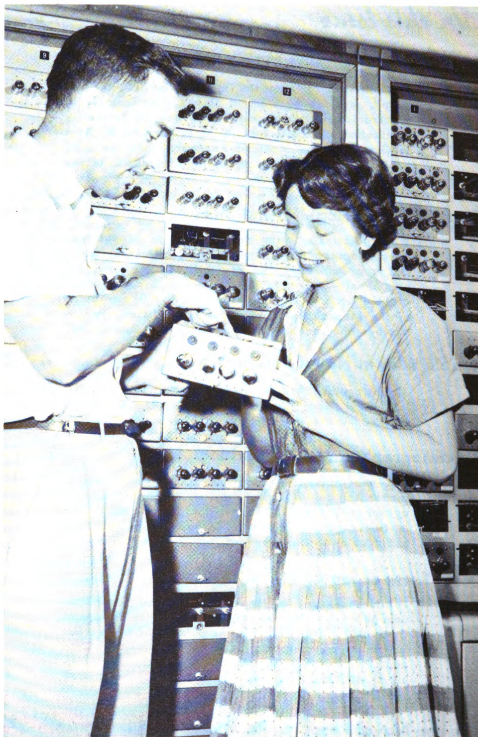
Two employees of the Naval Research Laboratory, Hester Snee and James Seward, inspect the workings of an electronic digital computer which has approximately 600 plug-in units. When something goes wrong with one of them it can be removed as easily as a bureau drawer and repairs can be made without extensive rewiring. This is only one of the ways in which unitization can be used to minimize electronics maintenance.
