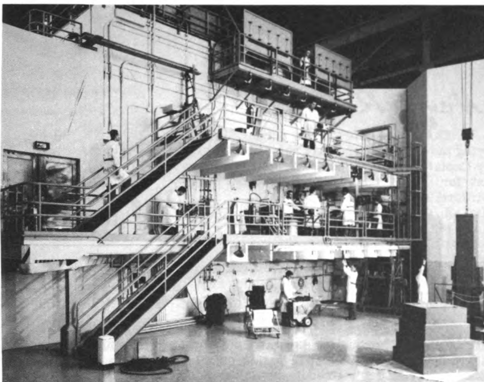
West face of the Brookhaven nuclear reactor. The steel and concrete plug in the right foreground is used to seal off openings in the top of the reactor. The facility for treating patients is on top and cannot be seen.
