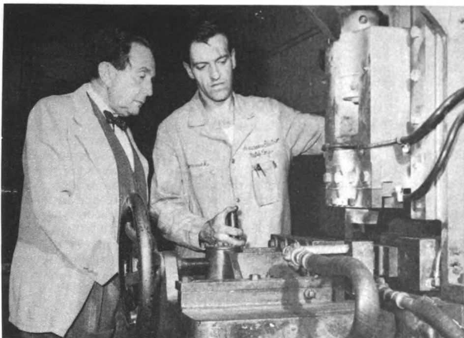
An early stage of powder metallurgy is pressing the metal powder. Here, Dr. Schwarzkopf and an assistant are watching the operation of the press.
