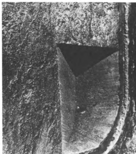
Phenolic foam-filled blister void with section removed to show completeness of filling
