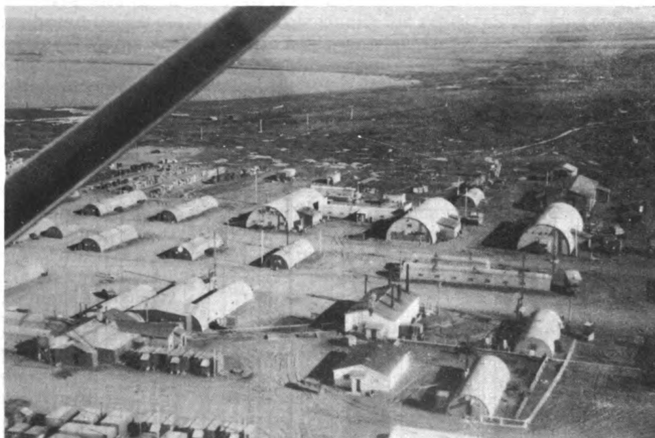
Figure 1 - ARL is the H-shaped building in the center.
