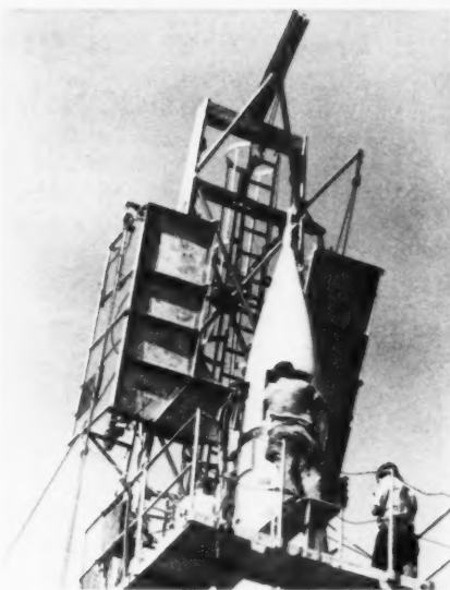
Figure 8 - Men working on instrumentation head section of VIKING No. 4 later launched from USS NORTON SOUND.
